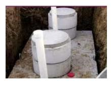
Prior to leak testing the septic tank, ensure that all risers and cleanouts are installed to the proper grade and sealed with grout or tar. The water level for the leak test should be filled to a point 10 cm above the highest level where a pipe or riser enters or attaches to the tank.
