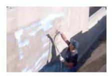
Worker prepares the surface of a concrete structure for waterproofing. It involves scraping off loose materials and paint, and ensuring there is a clean and dry surface for applying the waterproofing materials.
